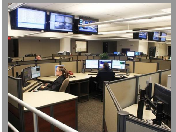
SPD Telecommunications Center
